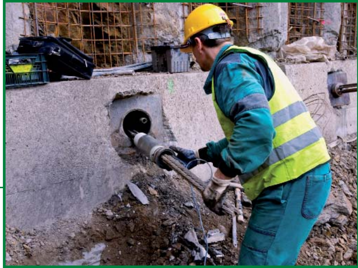
Sensor installation on ground anchor
