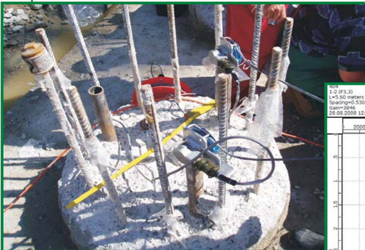
measurement of the integrity of piles using CHA apparatus
