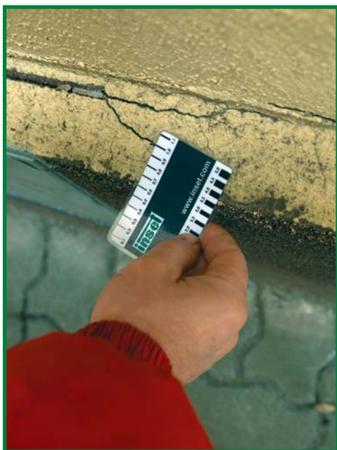
use of orientation gauges to determine the distribution of fractures
