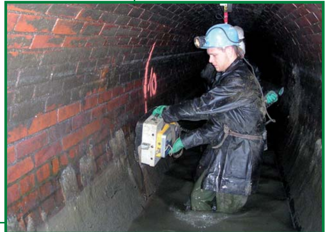
ground-penetrating radar investigation from the conduit
