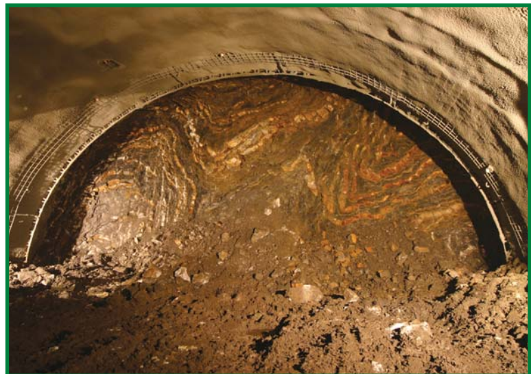
geological monitoring and documentation of the working face
